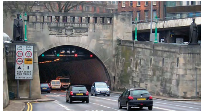
Northern portal to the Queensway Tunnel in Liverpool. Note the four lanes of traffic with no central barrier. Also visible are statues of King George V and Queen Mary on either side of the tunnel entrance, as well as the original street lights
